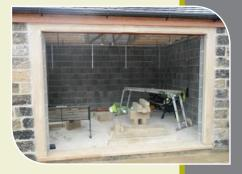
**Step 3** – Suitable xings should be used to secure the frame positioning 150mm to 250mm from each corner, then at a maximum of 600mm centres thereafter. Adequate support should be positioned between the brickwork and frame to prevent distortion when tightening the fixings.
