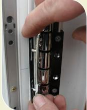
**Step 13** – Compression adjustment can be made by rotating the cap at the end of the shoot bolts. Loosen the lockingscrew rst then lock o once adjusted.
