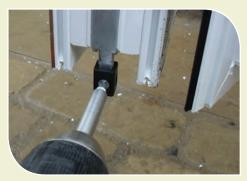
**Step 14** – Any final adjustment then can be made to the bottom roller wheels position then lock o the grub screw.
