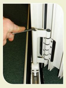
**Step 10** – Top rollers should be adjusted to maintain compression/contact against the track.
