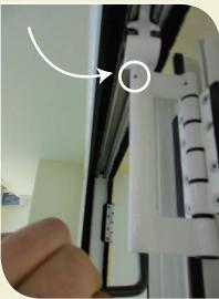
**Step 11** – Commence glazing starting with the first hinged door onto the frame. Each unit should be 'toe and heeled'.
