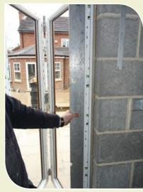
**Step 6** – The frame head should then be xed ensuring that it is parallel with the cill, again without twist and distortion. This can be aided by the use of a timber 'lat' or similar, cut to the internal height of the frame rebate and positioned along the width as a guide whilst fixing the head.
