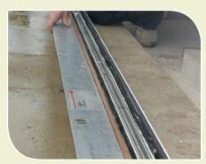
Silicone sealant should be applied to the drilled holes on the frame cill before the xings are inserted to prevent water seepage.
